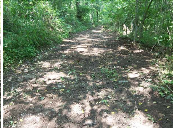
Road after repairs & grading
